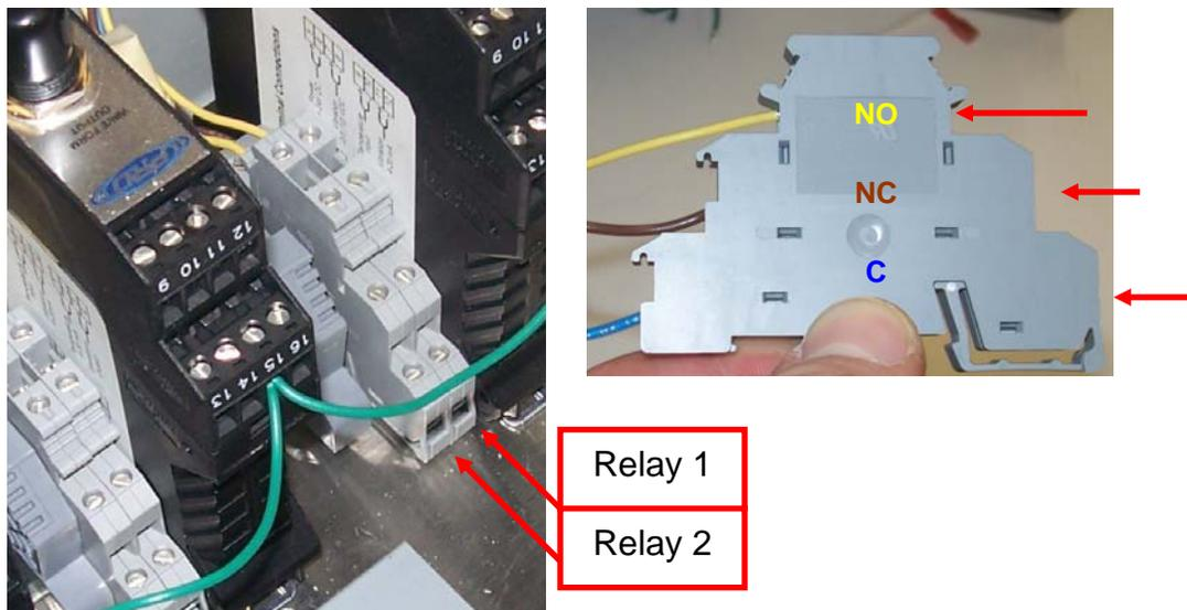
**Figure 6 – Relay Wiring**
